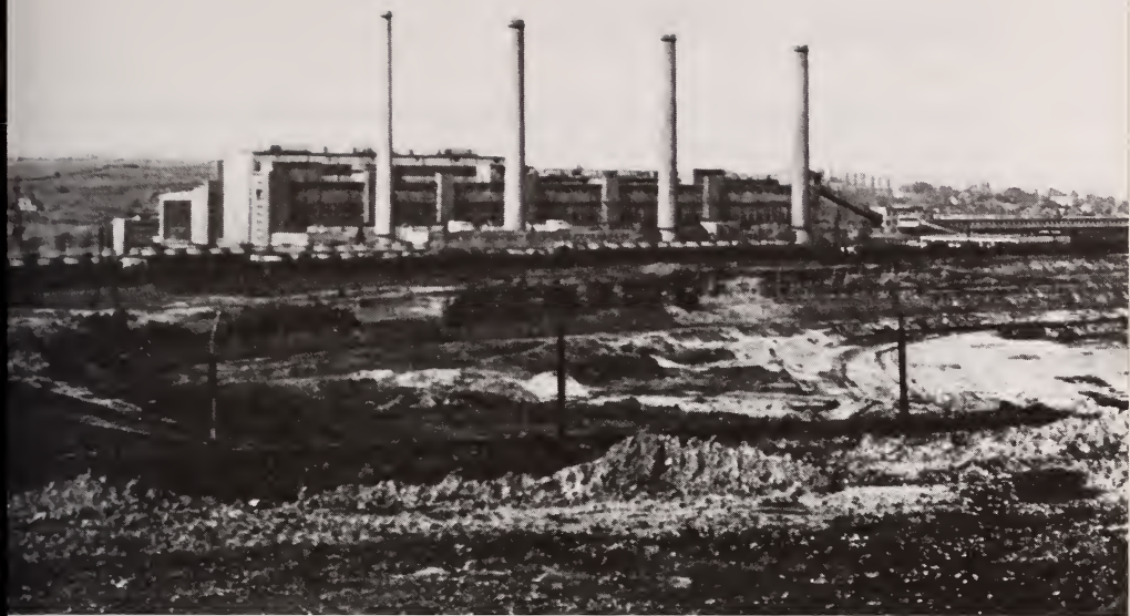
The Tisová power station, near Sokolov
