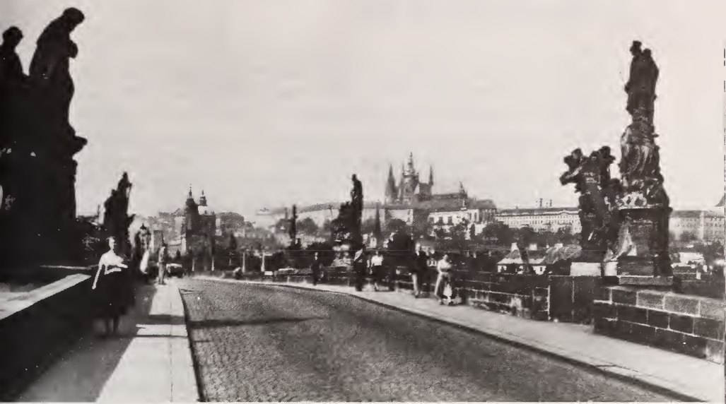
Charles Bridge, Prague
